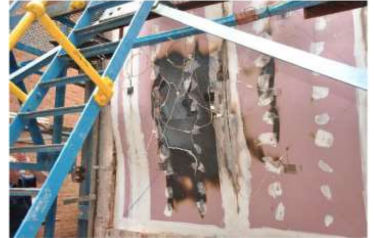
Figure 1.1: The unexposed side of the system after the test conclusion
